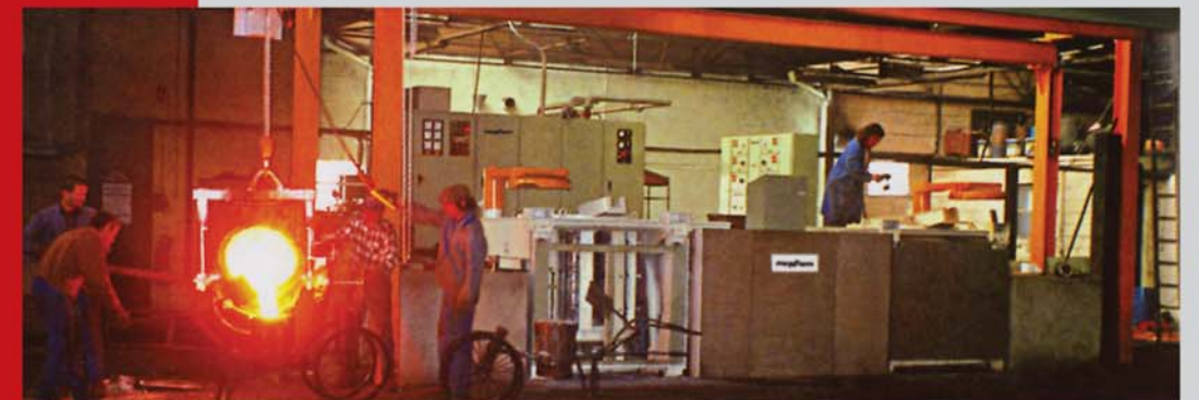
750kW, 1000Hz, 750KG Iron Melting Furnace in operation at F.A.C., Chatelleraut, France
